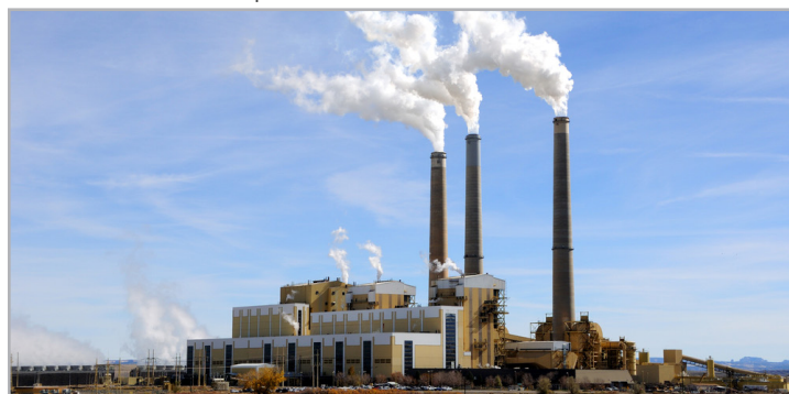
Fig. 2 Coal-fired power plant
