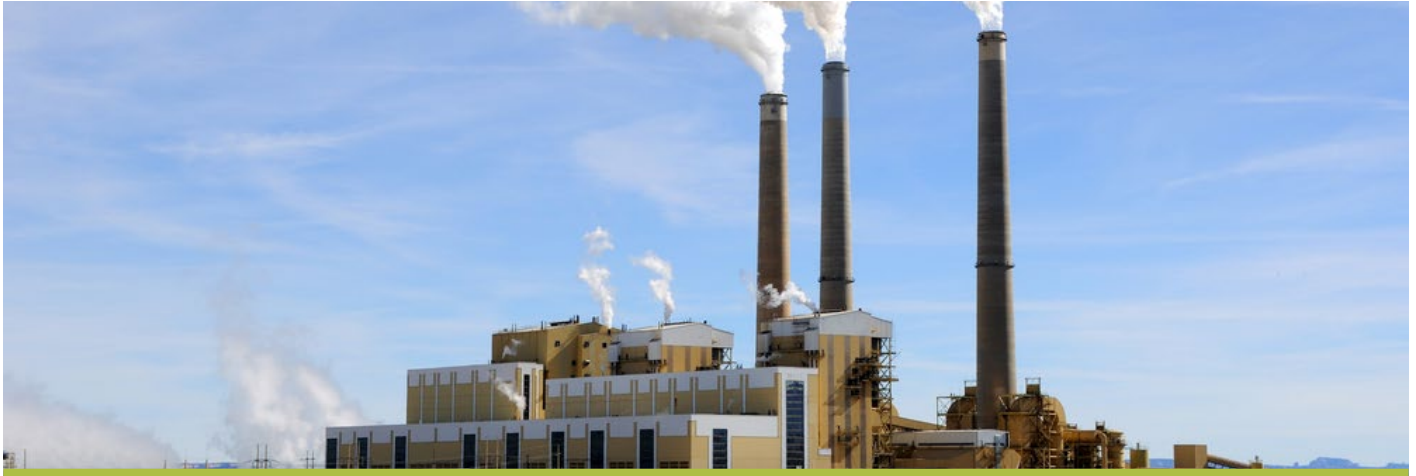
Fig. 2 Coal-fired power plant
